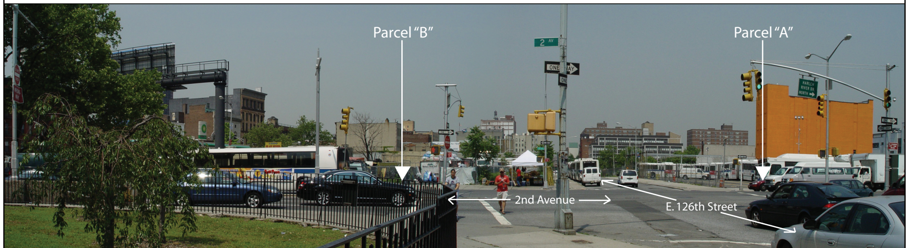
Viewpoint 32 - View of site (Parcel A & B) looking northwest from intersection of East 125th Street and Second Avenue
