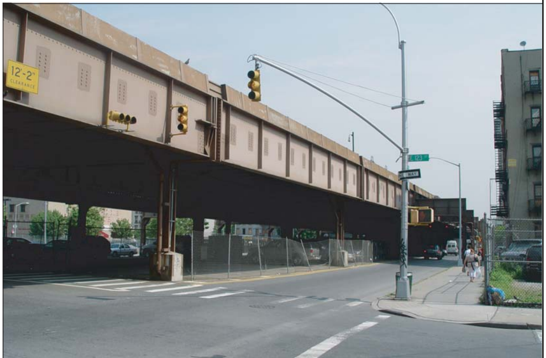
Viewpoint 10 - Metro-North Railroad Viaduct; view from E 123rd Street & Park Avenue
