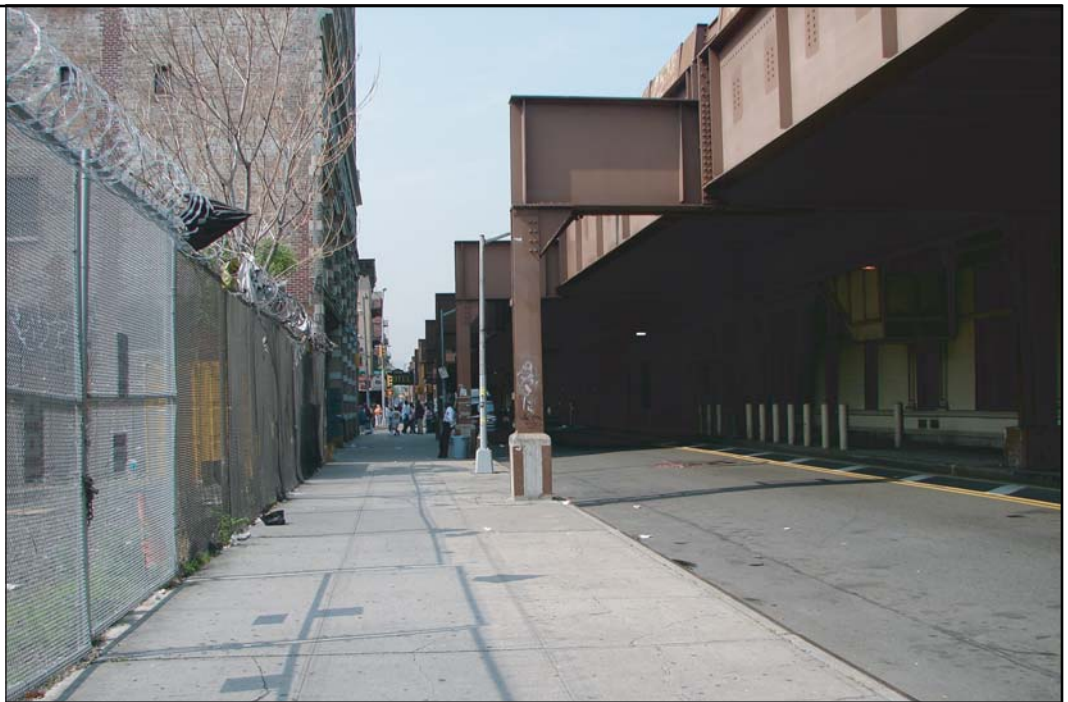
Viewpoint 9 - View of Metro-North Railroad Viaduct from street level
