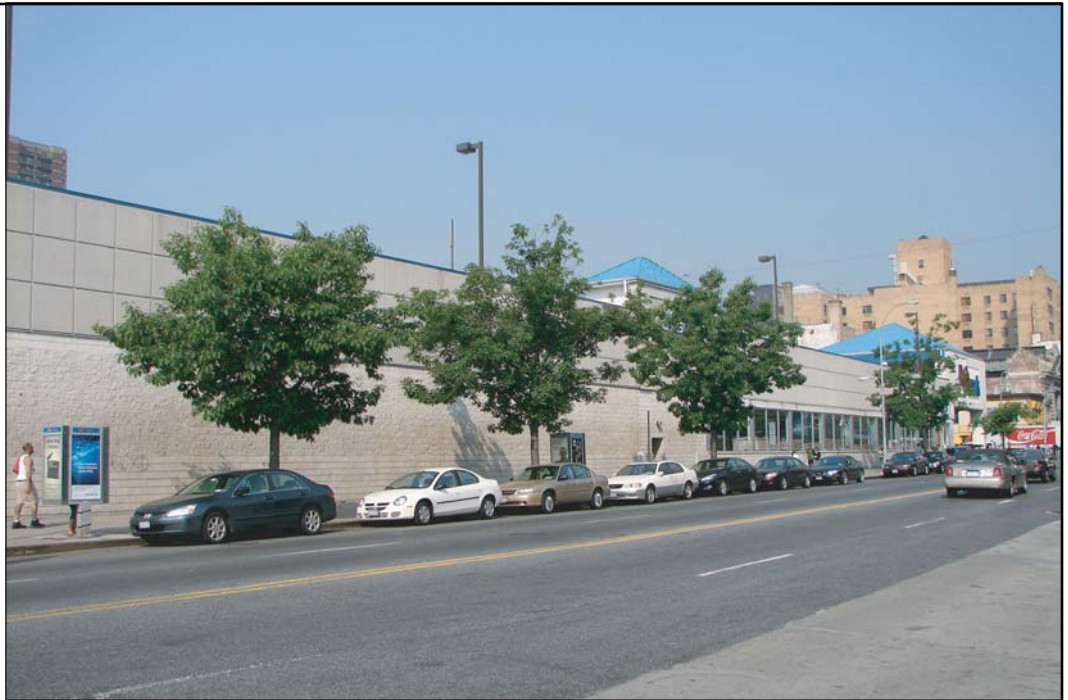
Viewpoint 14 - View of Pathmark building looking west between Third & Lexington Avenue
