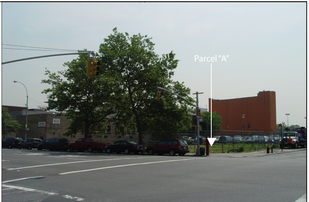
Viewpoint 33 - View of site (parcel "A") looking east from 126th Street & Third Avenue
