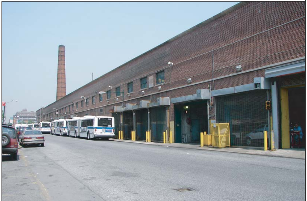
Viewpoint 30 - View of the MTA bus depot from First Avenue & E 125th St. intersection
