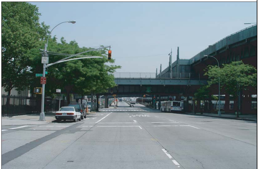
Viewpoint 28 - View looking north on First Avenue to Triborough Bridge ramps
